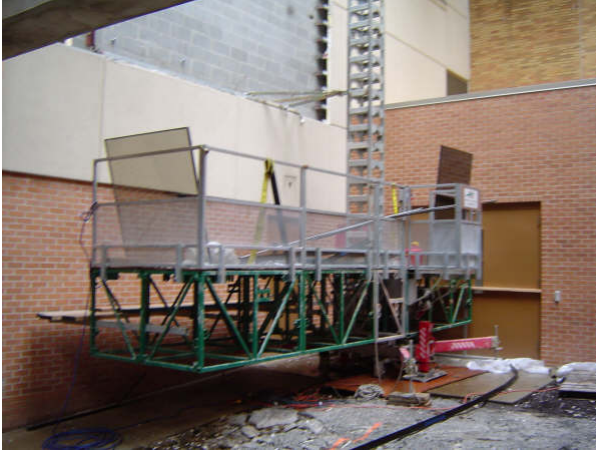
Figure 11 - Self Climbing Scaffold
