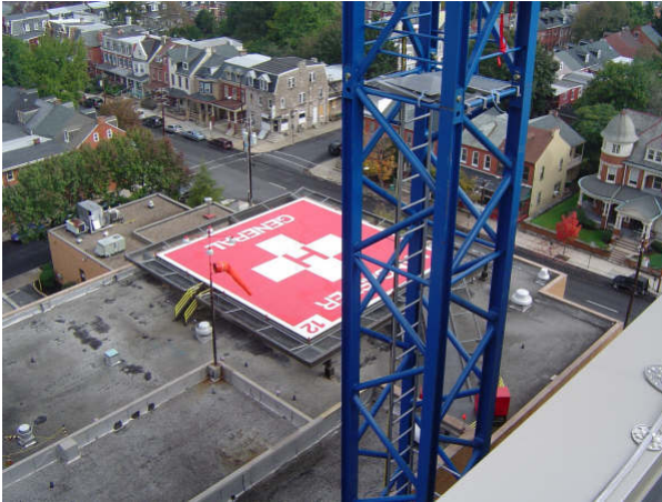
Figure 6 - Tower Crane w/ Helicopter Pad
