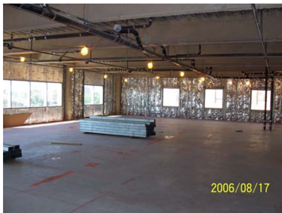
Figure 1 – 6 th Floor Shell Space
