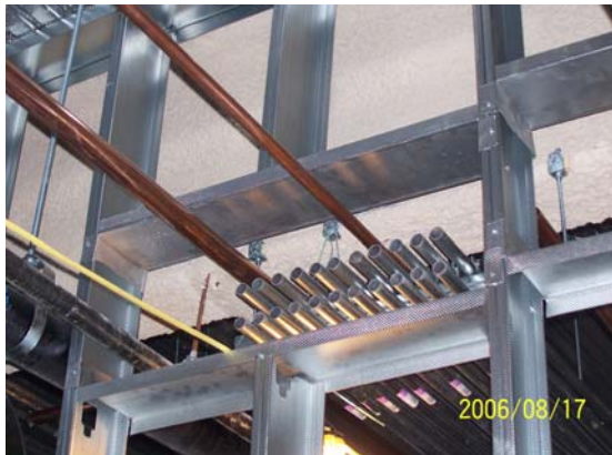
Figure 2 – 5 th Floor MEP Rough-in
