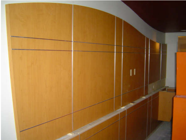
Figure 4 – 5 th Floor Patient Room Finishes
